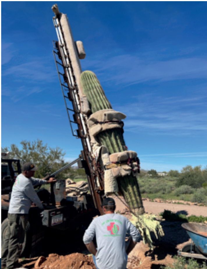
Crews replanting a mature saguaro cactus in our Box Canyon community
